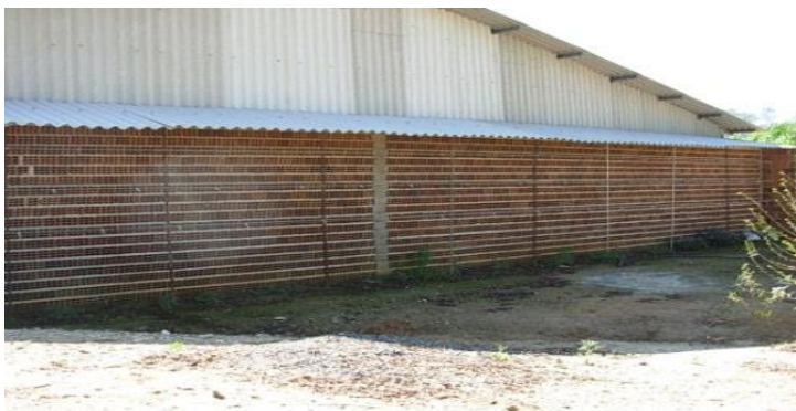
Figure 2 Porous wall (inlet)
